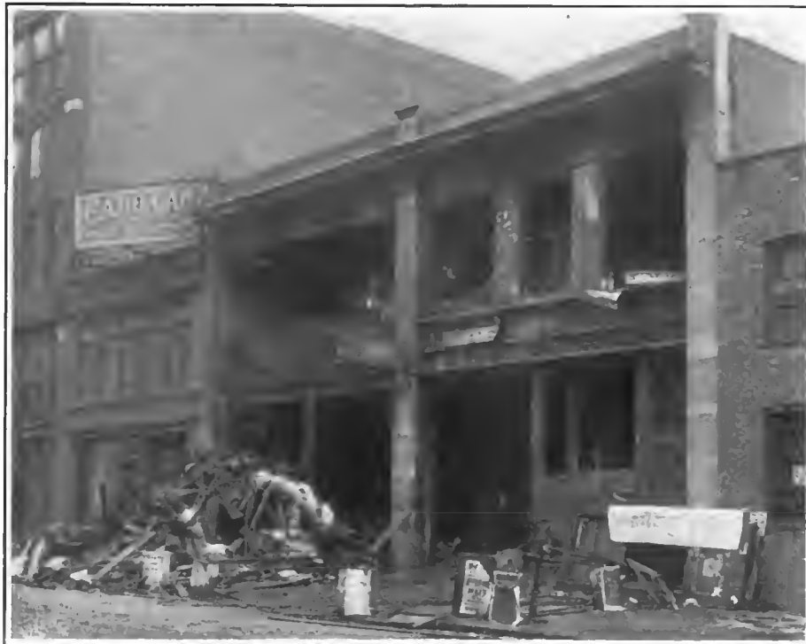
FRONT OF STANDARD GARAGE IN NEW YORK AFTER FIRE LAST WEEK.
